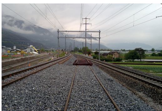
Fig. 24 - km 155,650, LEM630 provvisoria - Attività preparatorie per la connessione del binario 400 LEM630 provv./def. (in primo piano) al binario 400 Linea LE630 (a destra). Fig. 24 - km 155,650, temporary LEM630 - Preparatory activities for the connection with track 400 temp./perm. LEM630 (foreground) to track 400 of LE630 line (on the right).
