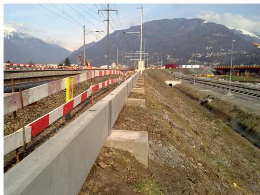
Fig. 17 - km 155,850, lato bin. 300 LEM630 definitiva - Ritenuta ghiaia definitiva con lastre prefabbricate in calcestruzzo. Fig. 17 - km 155,850, track 300 side, permanent LEM630 - Permanent ballast retainment with prefabricated concrete slabs.
