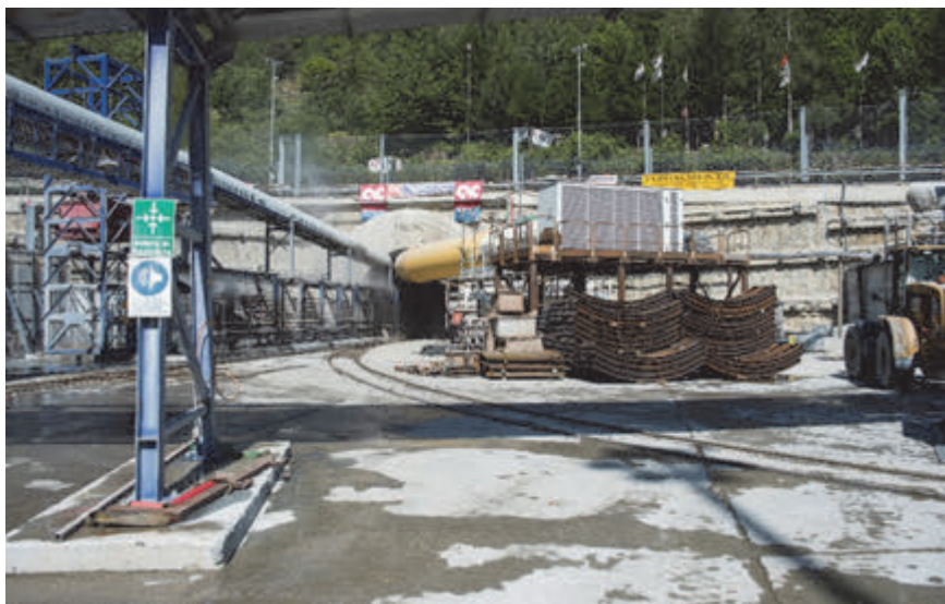
(Fonte: Tunnel Euralpin, Lyon Turin)
