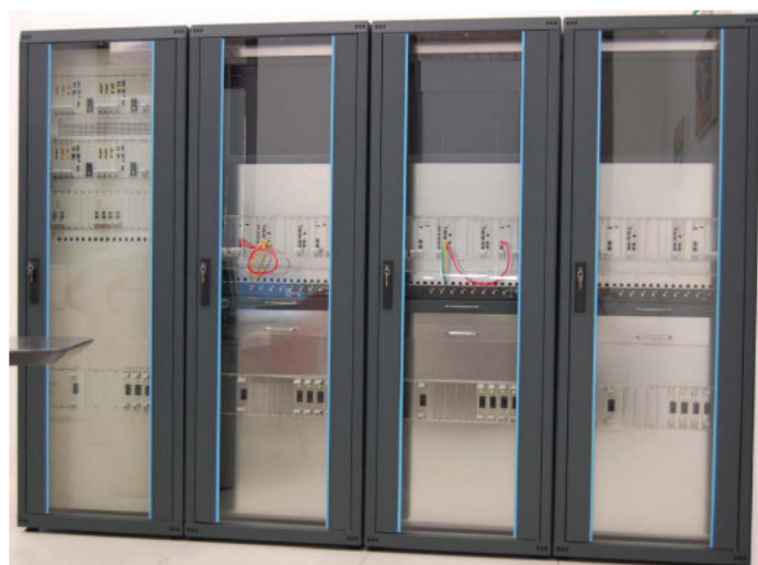
Fig. 9 - Elettronica del posto centrale ACC; da sinistra: il nucleo in sicurezza, i due armadi ART (normale e riserva) e l'armadio TEL. Electronics of the ACC Central Post; from left: the safety nucleus rack, the two ART racks (normal and backup), the TEL rack.
