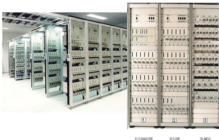
Fig. 12 - Posto periferico ACC Ansaldo STS. ACC peripheral post by Ansaldo STS (CDA/CDE = Area Controller/Field Controllers; MDC = Adaptation Units).
