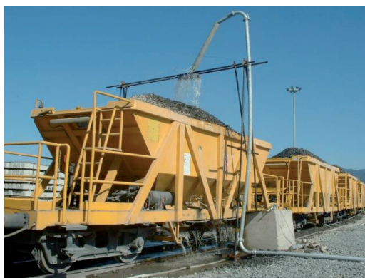
Fig. 17 - Cantiere CAR1. Impianto di lavaggio ballast. Construction yard CAR1. Ballast washing plant.
