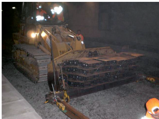
Fig. 19 - Posa del binario. Particolare sfilamento rotaie. Track laying. Detail of the extraction of the rails.
