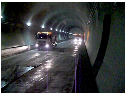
Fig. 11 - Galleria Firenzezuola. Formazione primo strato di ballast. Camion carico in retromarcia (sx) e camion scarico in normale senso di marcia (dx). Firenzezuola Tunnel. Formation of the first ballast layer. Loaded truck in reverse running (left) and unloaded truck in normal running mode (right).
