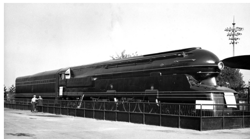
(Fonte - Source: Pennsylvania Railroad Photographs, < http://www.billspearsphotos.com/ > (Ultima consultazione - Last consultation: 03.08.2010).
