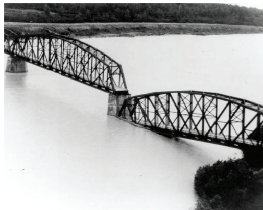
Fig. 2 - Il collasso del ponte Million Dollar in Alaska (1964). The Million Dollar bridge collapse in Alaska (1964).
