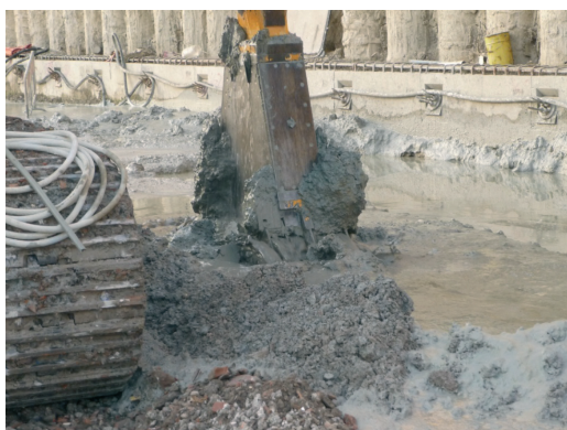
Fig. 27 - La fresa in azione. The milling cutter in operation.
