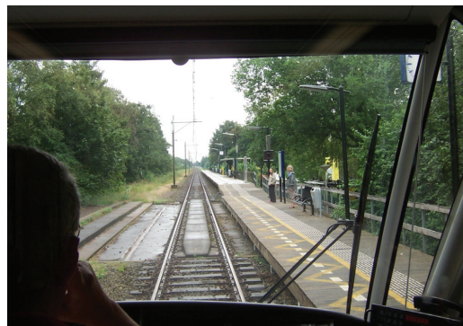
Fig. 6 - Banchina tram-treno in serie a una banchina ferroviaria alta, sporgente in senso orizzontale, presso RijnGouwelLijn (Olanda). Tram-train low platform in series with a railway high one, protruding horizontally, in RijnGouwelLijn (The Netherlands).
