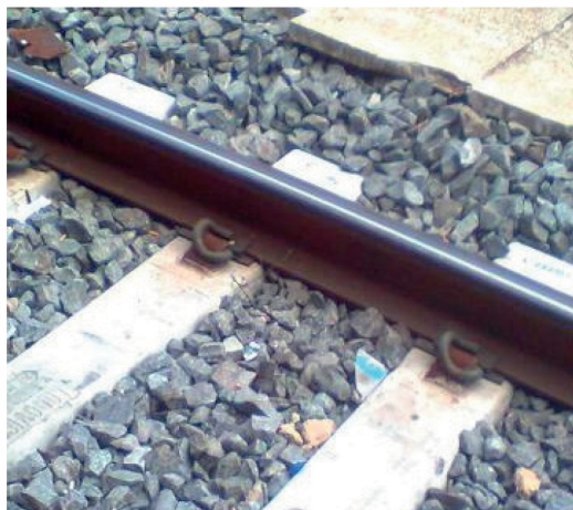
Fig. 26 - Traversa RFI 230 P - Attacco Pandrol. RFI 230 P sleepers - Pandrol fastening
