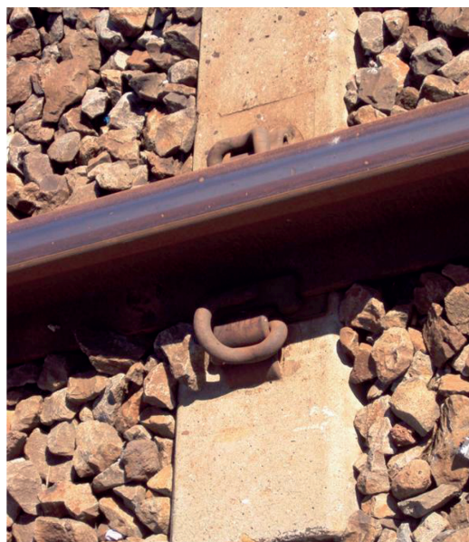
Fig. 16 – Traversa FS V 35 P – Attacco Pandrol. FS V 35 P – Pandrol fastening.
