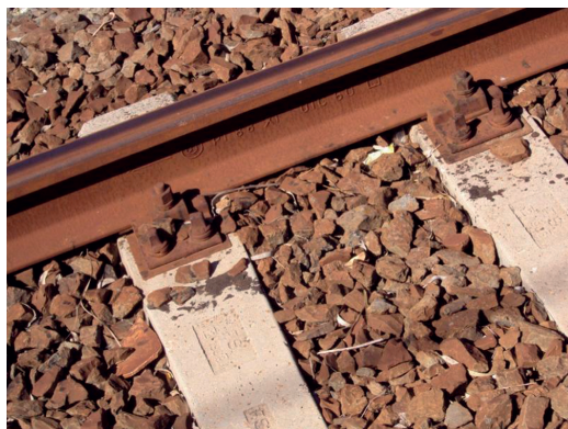
Fig. 14 – Traversa in cap FS V 35 – Attacco K – Piastra a 4 caviglie. FS V 35 Pre-stressed reinforced concrete sleeper – K fastening – Plate with 4 sleeper screws.
