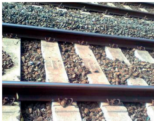
Fig. 27 – Traversa RFI 230 V – Attacco Vosloh. RFI 230 V sleeper - Vosloh fastening.
