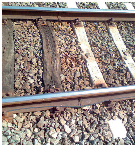
Fig. 19 - Traversa in cap M 62 - Attacco K - Piastra a 2 caviglie. M 62 pre-stressed reinforced concrete sleeper - K fastening - Plate with 2 sleeper crews.
