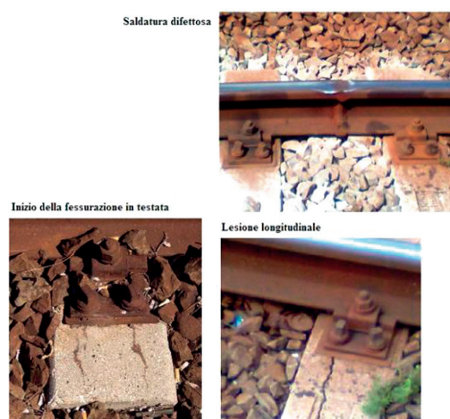
Fig. 30 - Lesioni in traverse in cap. Damages in precompressed reinforced concrete sleepers.
