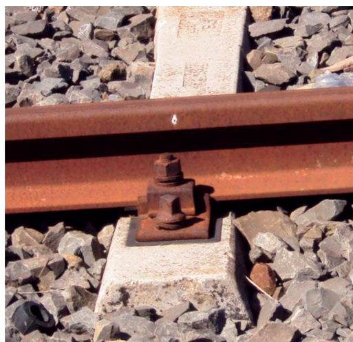
Fig. 7 – Traversa FS in esercizio – Attacco K, piastra a 2 caviglie. FS sleeper in operation – K fastening, plate with 2 sleeper crews.
