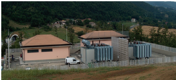
Fig. 8 – Nuova SSE di Idice con reparti AT ed MT blindati. New Idice substation with high-voltage and medium-voltage metal clad compartments.
